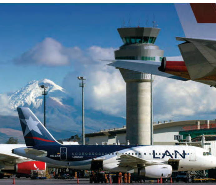
In 2003, OPIC committed $200 million in financing to support the construction of the Mariscal Sucre International Airport (Quiport) in Quito, Ecuador. Since opening in 2013, the airport has produced far-reaching benefits from Ecuador to the United States. (OPIC)
