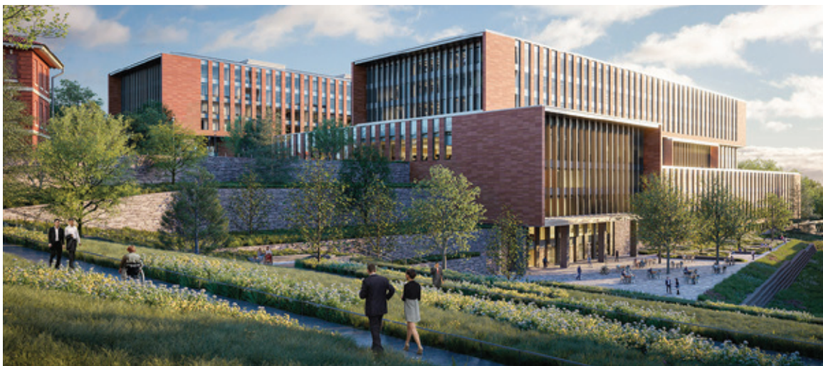
CAD design for new facility for Cybersecurity and Infrastructure Security Agency. Source: Government Services Agency
