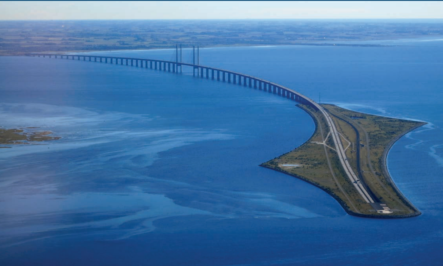
The Öresund or Øresund Bridge is a combined railway and motorway bridge across the Øresund strait between Denmark and Sweden. Image by: Nick-D (Wikimedia Commons). September 28, 2015
